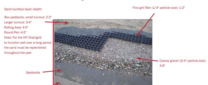
Undisturbed earth, capable of load-bearing; leveled to 1% gradient
